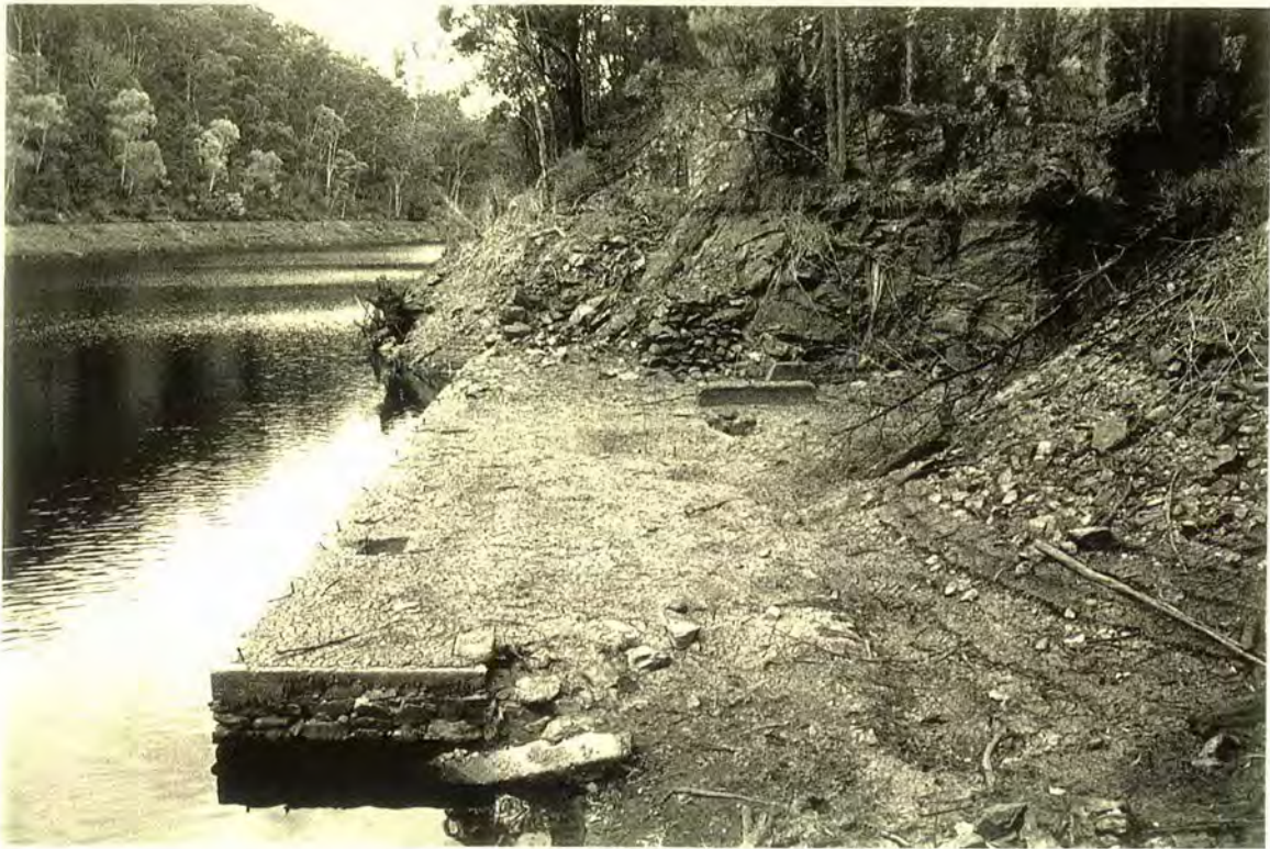
Figure 31. Pioneer processing plant, concrete platform, normally inundated
