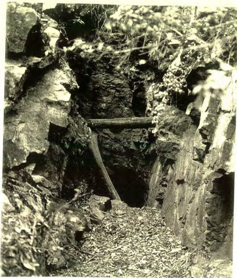
Figure 61. Caledonian workings, tunnel
