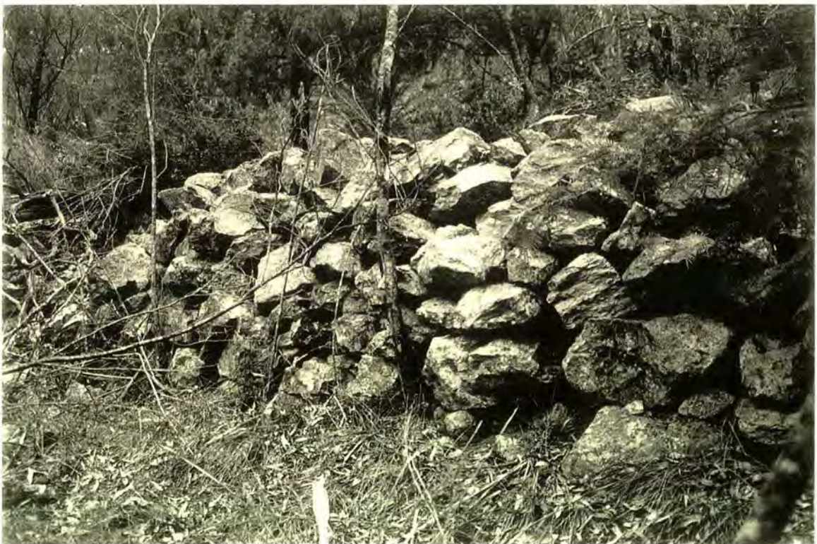
Figure 66. Embankments near Black Lode
