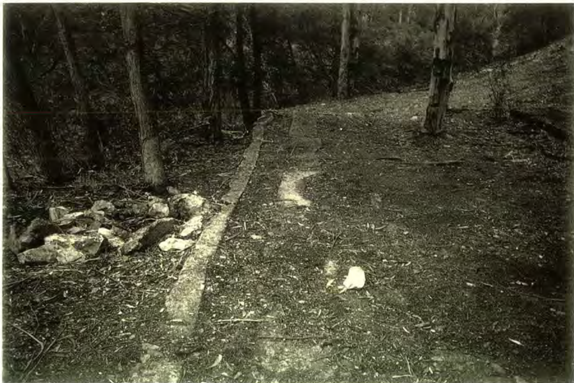
Figure 34. Homeward Bound processing plant, concrete foundations, facing north
