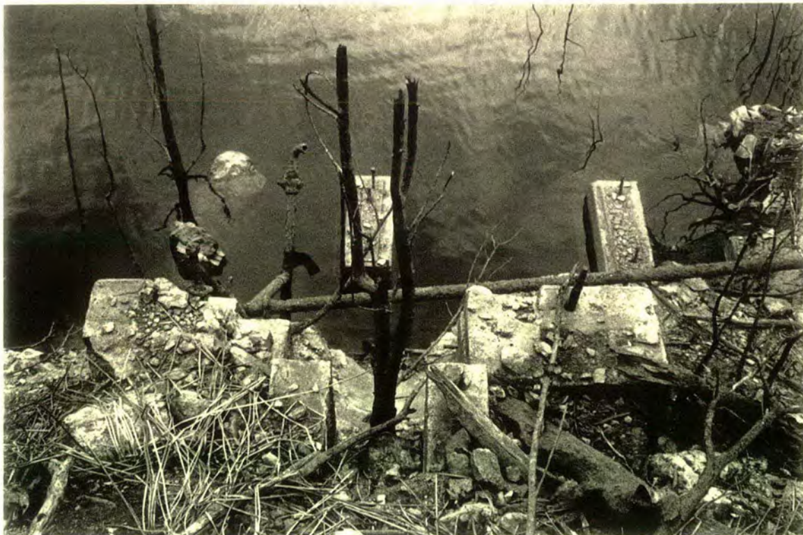
Figure 16. Golden Crown processing site, concrete spillway or chute looking towards concrete blocks for stamp site (normally under water)
