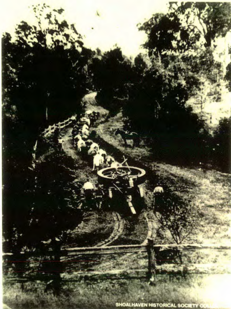
Figure 7. Hauling fly wheel up Danjera Gap road (Nowra and District Historical Society)
