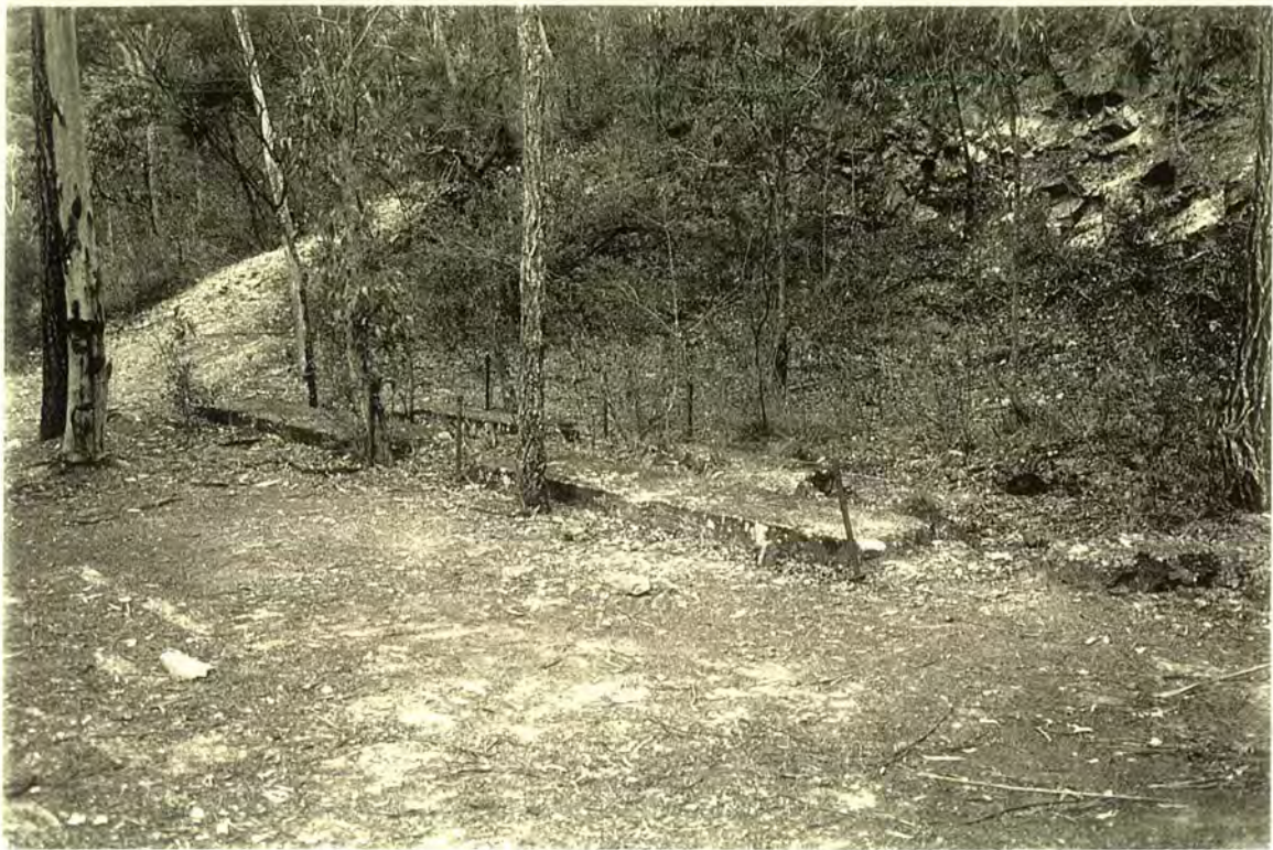
Figure 33. Homeward Bound processing plant, concrete area, site for 40 head stamps
