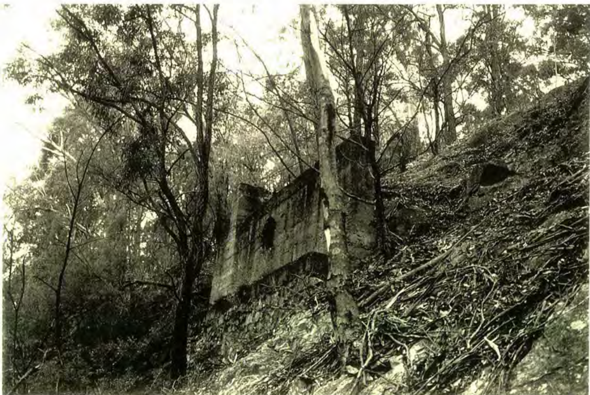
Figure 30. Pioneer processing plant, chute
