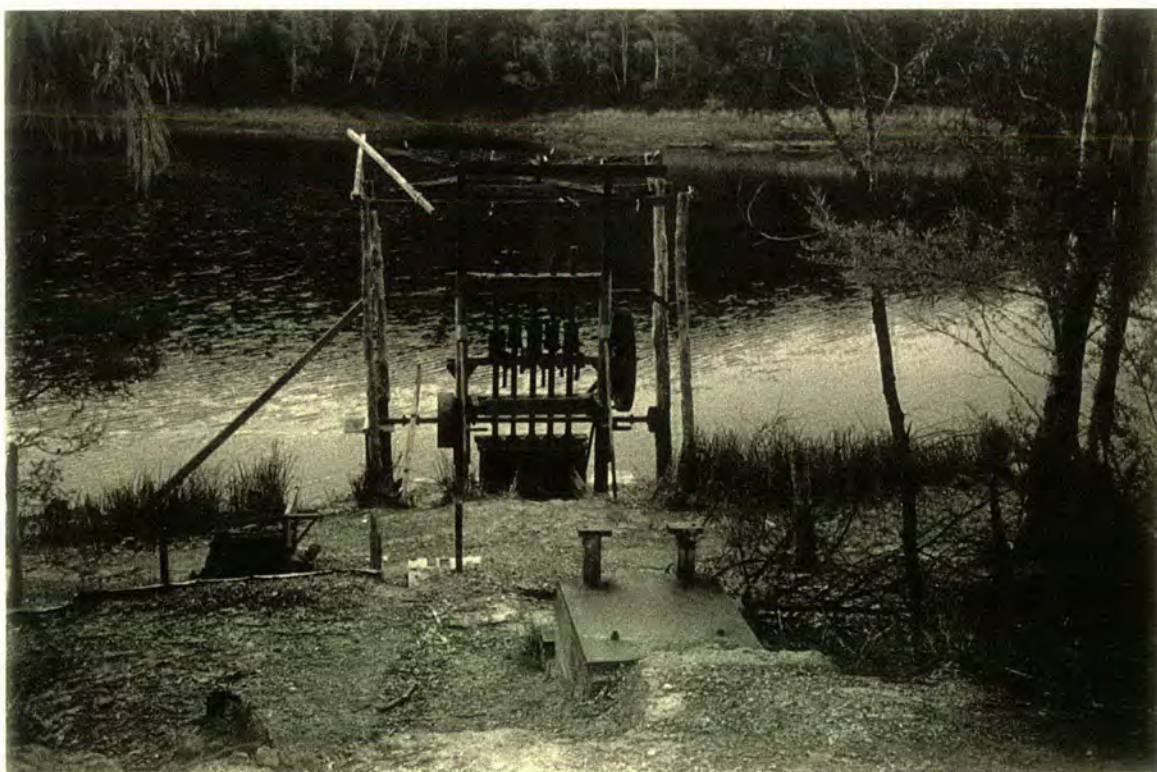
Figure 12. Chapman's battery, looking north
