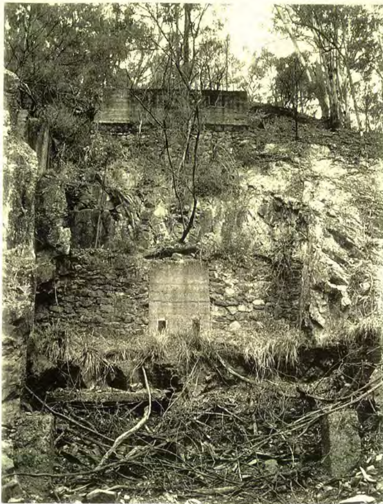
Figure 29. Pioneer processing plant, back end of site
