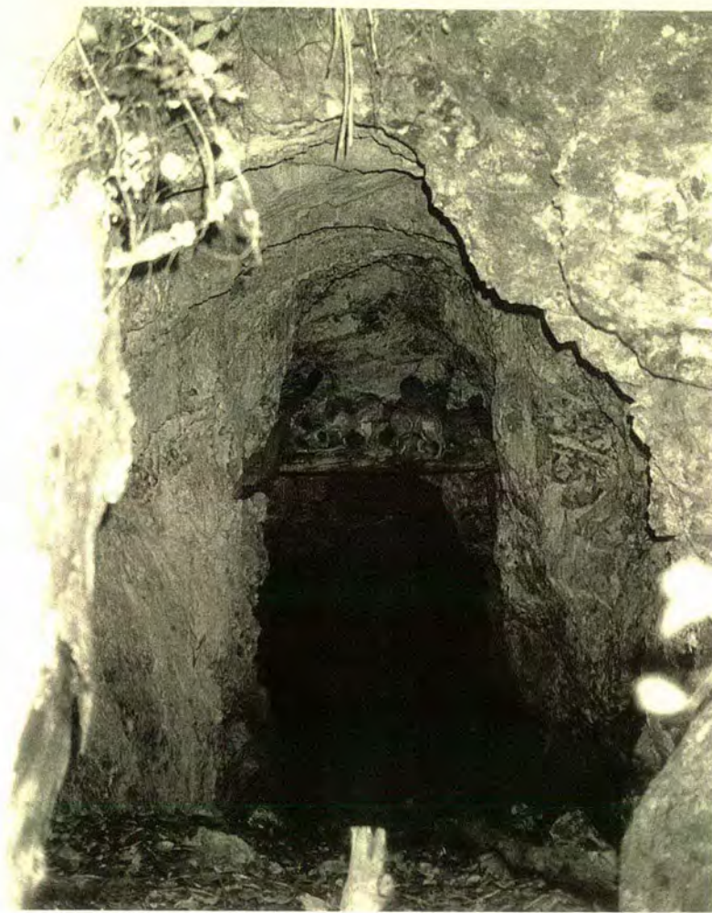
Figure 63. Golden Quarry No 3 adit
