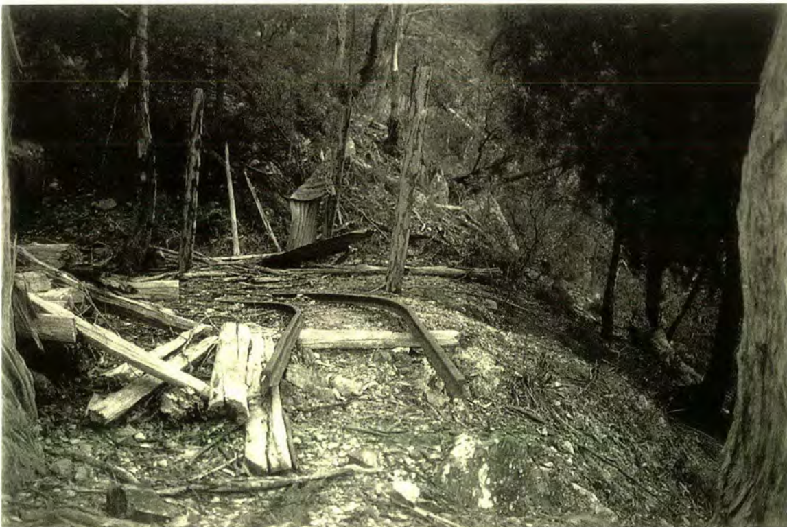
Figure 38. Homeward Bound lower tunnel, tramway
