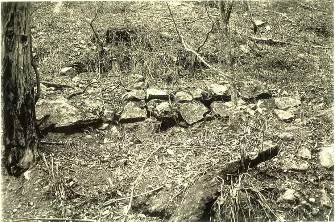
Figure 65. Pioneer tramway, north of main track near Black Lode
