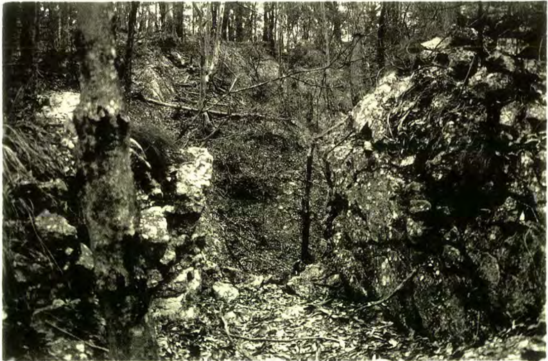
Figure 54. Culvert entrance to Pioneer No 2 quarry, facing south
