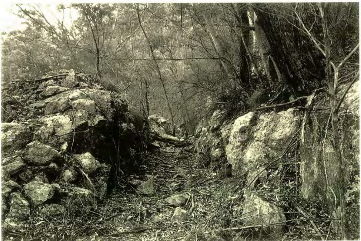
Figure 56. Tramway culvert near Pioneer No 2 quarry, facing south east
