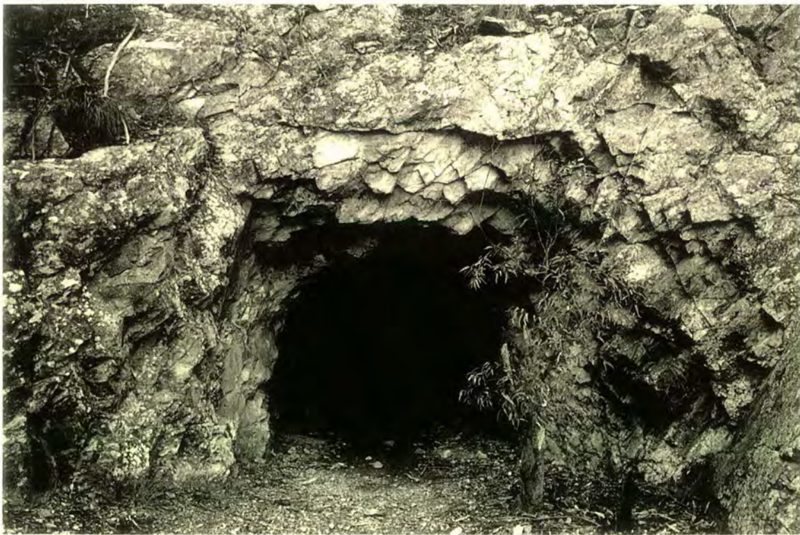
Figure 40. Homeward Bound upper tunnel, west entrance
